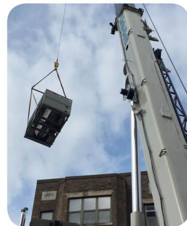
The new chiller was lifted by crane to the Kairos House roof.
